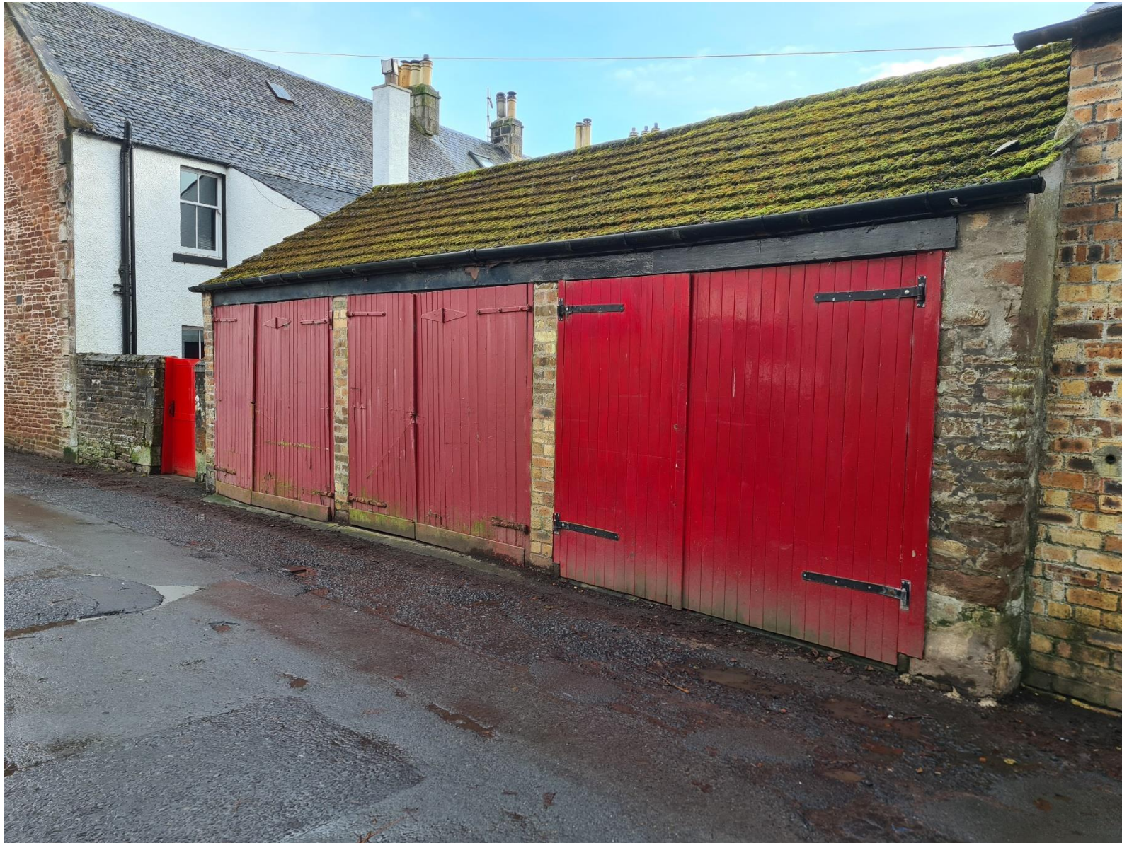
Fig 5: Photograph of vehicle doors serving the outbuildings of the Graham Institute, taken from Lower Green (adopted street) (Source: Mr & Mrs Barton).
